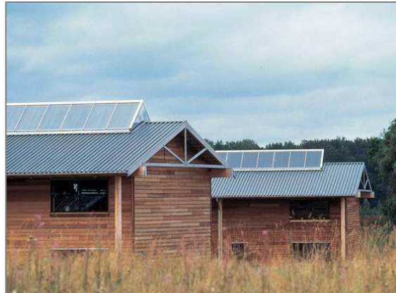
HAVREVANGEN 2: SOLAR PANELS
