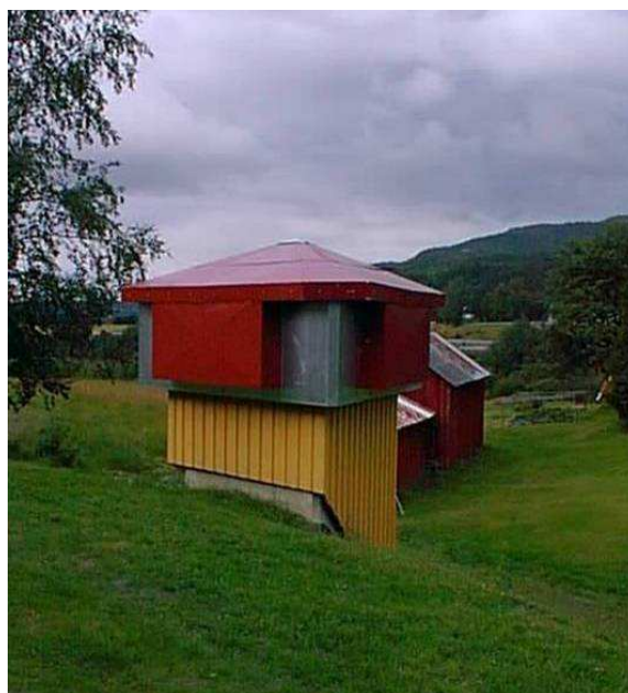
GRONG SCHOOL 4: AIR INLET TOWER
