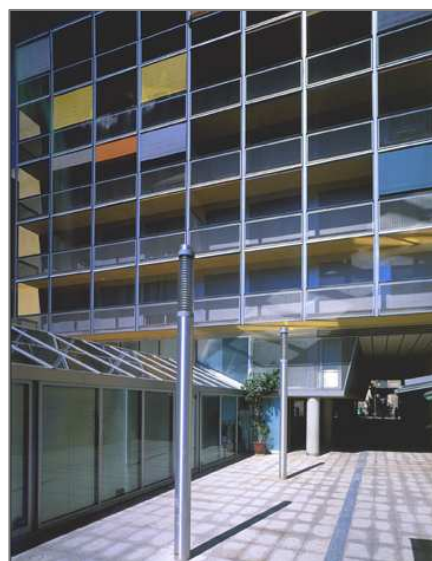
PAU CLARIS 2: SW FAÇADE'S GALLERIES
