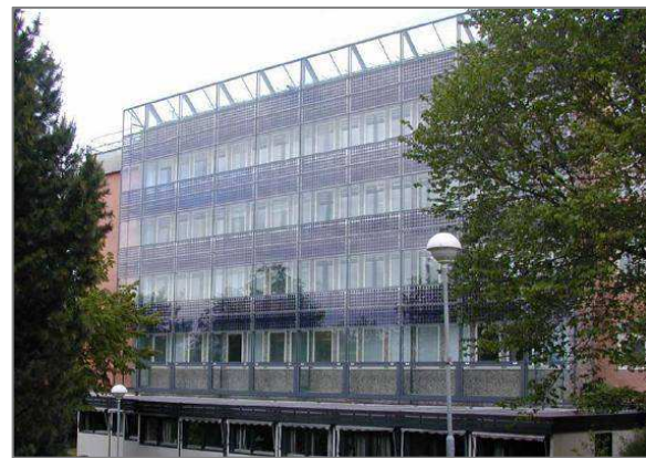
GLØSHAUGEN 1: FAÇADE BEFORE AND AFTER
