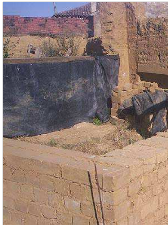
AMAYUELAS 2: ADOBE CONSTRUCTION
