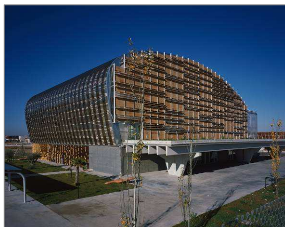
CALL CENTER 1: EXTERIOR VIEW
