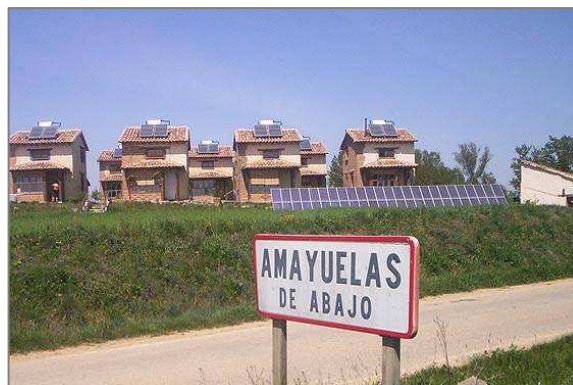
AMAYUELAS 1: GENERAL VIEW
