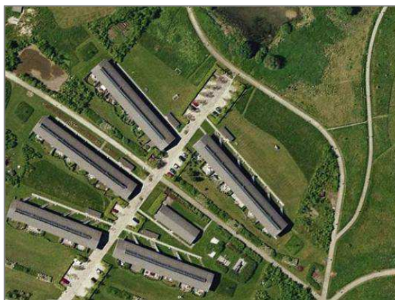
HAVREVANGEN 1: GENERAL VIEW
