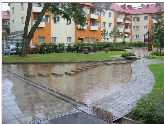
AUGUSTENBORG 4: STORMWATER SYSTEM
