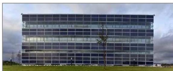
ACCIONA 1: SOUTH FAÇADE
