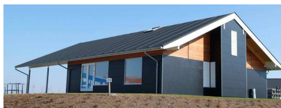
SEEST 1: GENERAL VIEW
