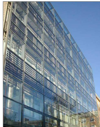
GLOSHAUGEN 3: FAÇADE INTEGRATED PV CELLS
