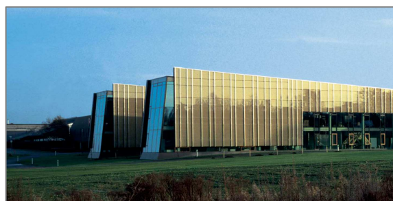
ROCKWOOL 1: GENERAL VIEW
