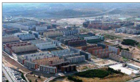
VALDESPARTERA 1: GENERAL VIEW
