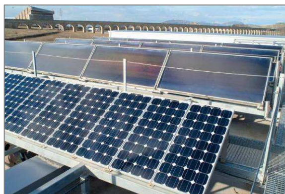
CENIFER 2: SOLAR AND PV PANELS
