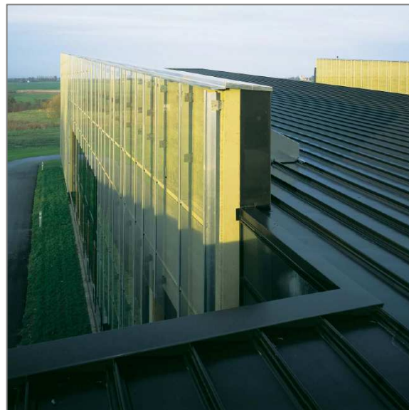
ROCKWOOL 2: WEST FAÇADE AND ROOF
