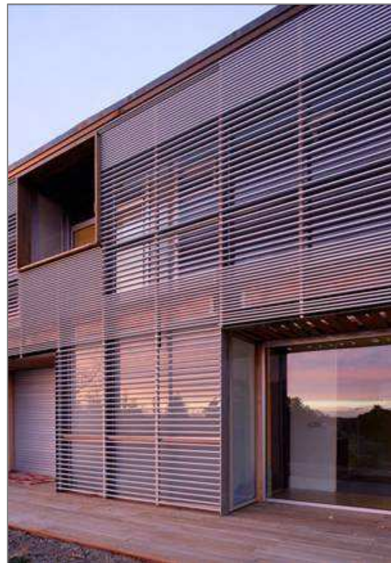
FUJY HOUSE 2: SOUTH FAÇADE DETAIL Integration of renewable energies in buildings and town planning
