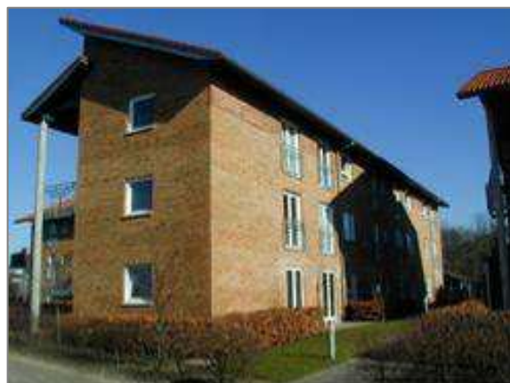
HERNING 2: RAINWATER IS COLLECTED
