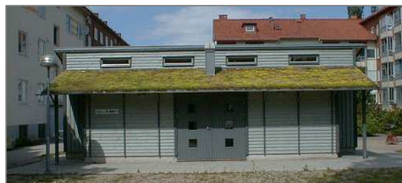
AUGUSTENBORG 5: RECYCLING CENTRE
